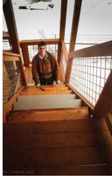
New construction at TwispWorks. Photo by Angela Ang.
